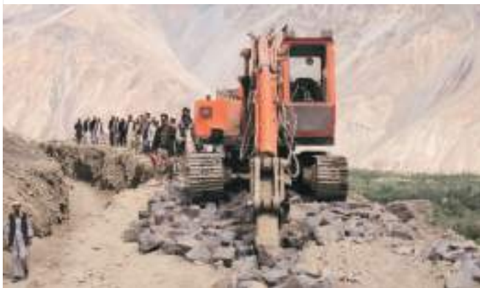
Micro-Hydel Water Channel Construction at Laspur Project Site
