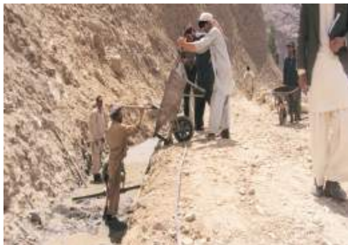
Micro-Hydel Water Channel Construction at Yarkhun Project Site
