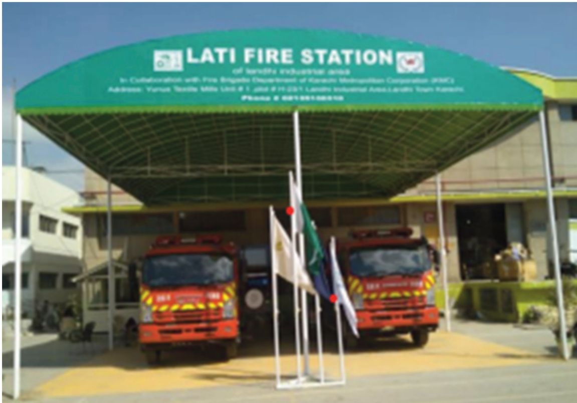
Fire Engines parked ready to take off in emergency response
