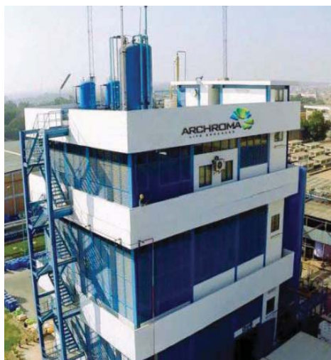
Liquid Indigo production facility at Jamshoro site
